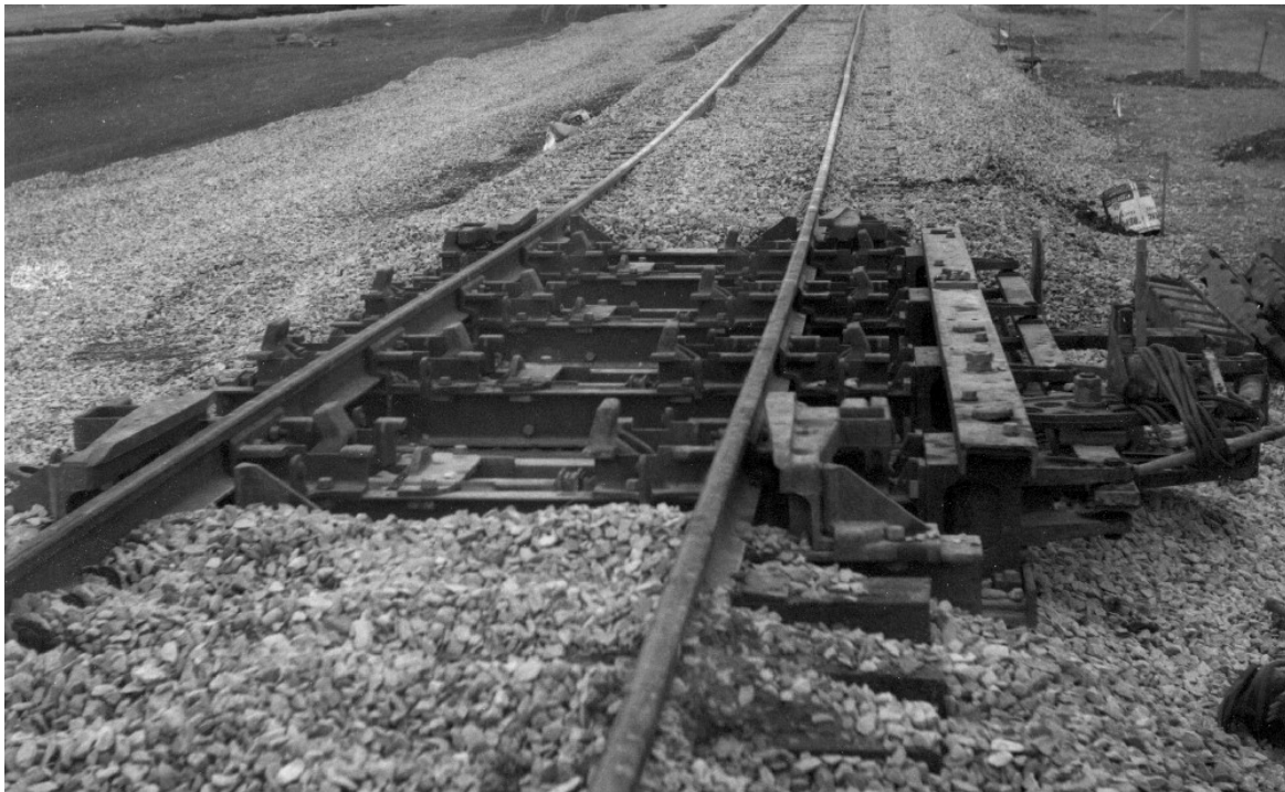
Retarder at Buckeye yard.
