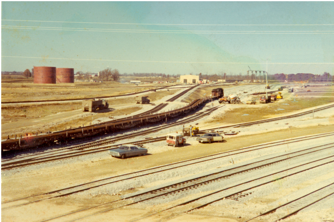
Photo taken from the hump looking at the two 1,000,000-gallon fuel tanks, the diesel service & repair shop, and the diesel fuel & sanding platform. A rail train looks ready to unload.
