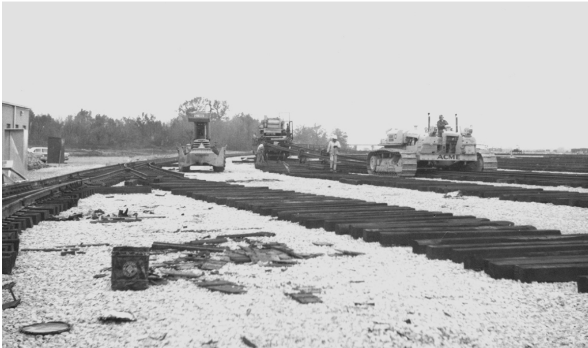
Track under construction at Buckeye Yard.
