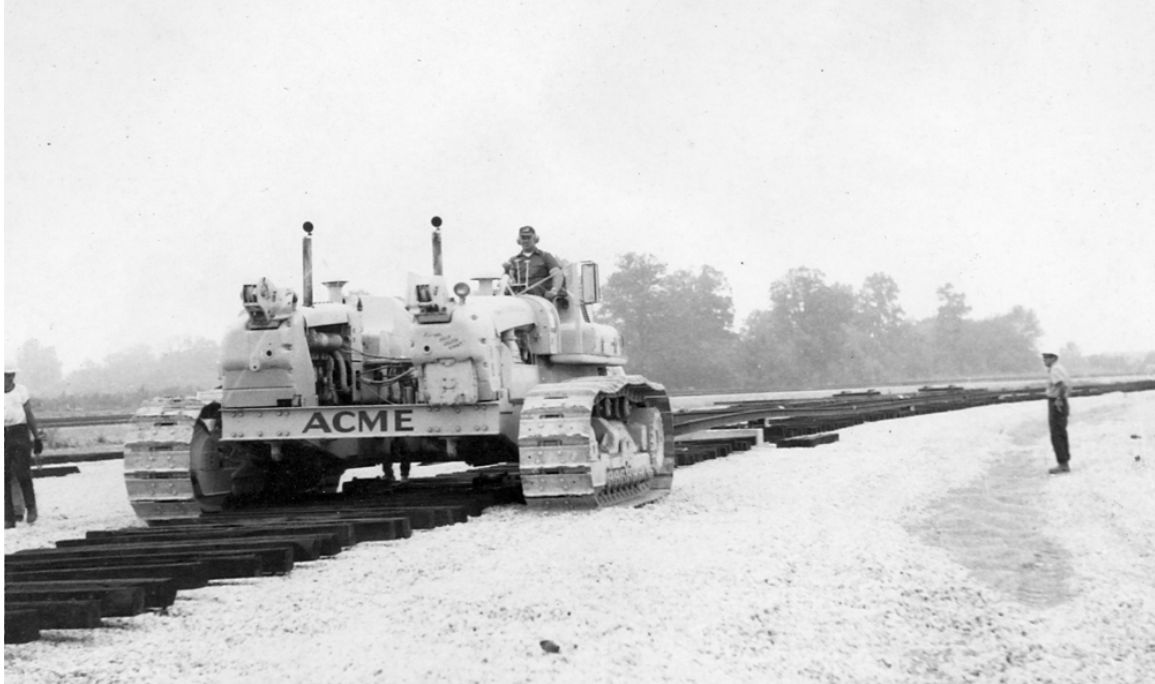
A dual engine crawler pulling rail.
